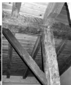
Reused barn beams in timber frame home
