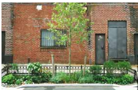
Right-of-way bioswales collect rainwater, reduce urban heat island effect, and improve air quality
